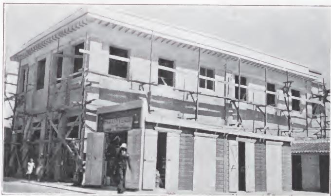
Office under construction for Banking and other Business Departments
